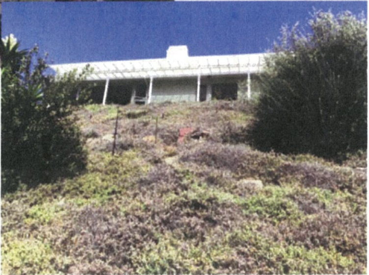
1569 Tahiti Ave Rear view (South side)
